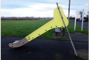
**Finding:** The tube(s) on this item have corroded from the inside and split the steel
